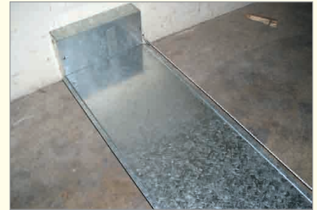
1. Mark the start point from the installation layout plan.
